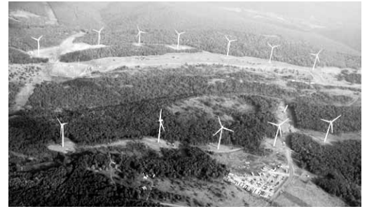
Part of the NedPower/Mount Storm wind facility in West Virginia. Photo: Bruce Halgren
