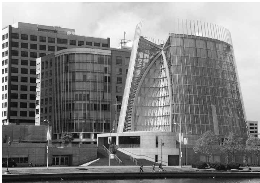
The glass panels comprising the exterior of the Cathedral of Christ the Light in Oakland, Calif. include patterns made of ceramic dots, or “frit.” The patterns contribute to the building’s extensive use of natural light in its interior, while also making it safe for birds. Photo by CTG/SF, flickr.com
