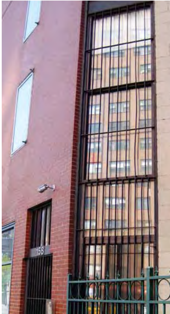
This security grille also creates a pattern that will deter birds from flying to reflections. Photo: Christine Sheppard, ABC
