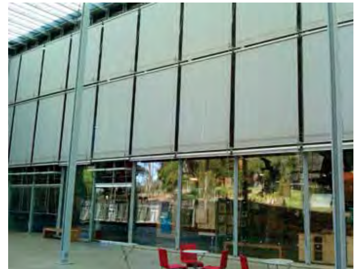
External shades on Renzo Piano's California Academy of Sciences in San Francisco are lowered during migration seasons to eliminate collisions. Photo: Mo Flannery
