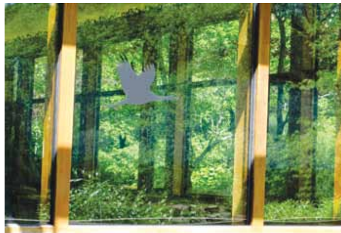
A single decal is minimally effective for collision prevention on a window of this size, as there is still a substantial amount of untreated glass. Photo: Christine Sheppard, ABC
