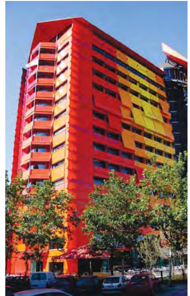
The Hotel Puerta America in Mexico City was designed by Jean Nouvel, and features external shades. This is a flexible strategy for sun control, as well as preventing collisions; shades can be lowered selectively when and where needed. Photo: Ramon Duran
