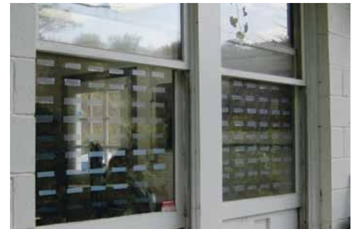
Tape decals (Window Alert shown here) placed following the 2 x 4 rule can be effective at deterring collisions. Photo: Christine Sheppard, ABC
