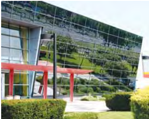
Reflections in this angled façade can be seen clearly over a long distance, and birds can approach the glass from any angle. Photo: Christine Sheppard, ABC
