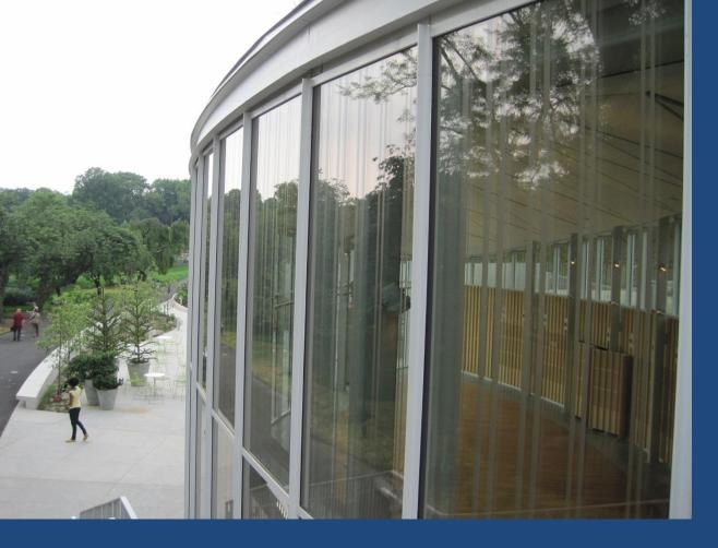
Situations like this one, where birds can see through a building, can be collision hazards. Here, the frit pattern on both glass walls is visible, reinforcing the 'do not fly' signal.
