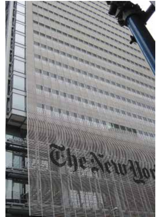
The façade of the New York Times building, by FXFOWLE and Renzo Piano, is composed of ceramic rods, spaced to let occupants see out while minimizing the extent of exposed glass—good for controlling heat and light, and safe for birds. Photo by Christine Sheppard, ABC
