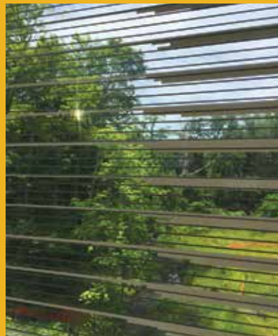
Glass detail, showing frit pattern
