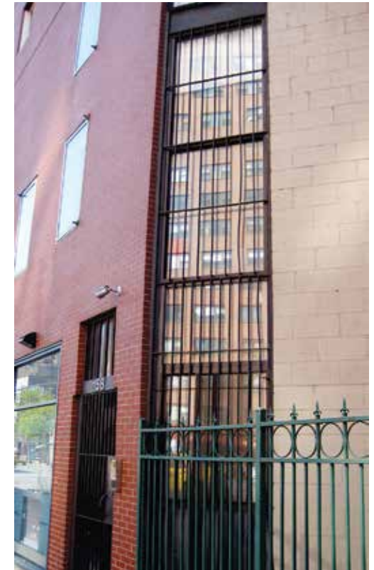
This security grille creates a pattern that will deter birds from flying to reflections. Photo by Christine Sheppard, ABC
