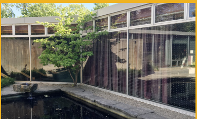
Feather Friendly Residential is applied as a tape, but the backing is removed, leaving a pattern of dots. Photo by Chris Early
