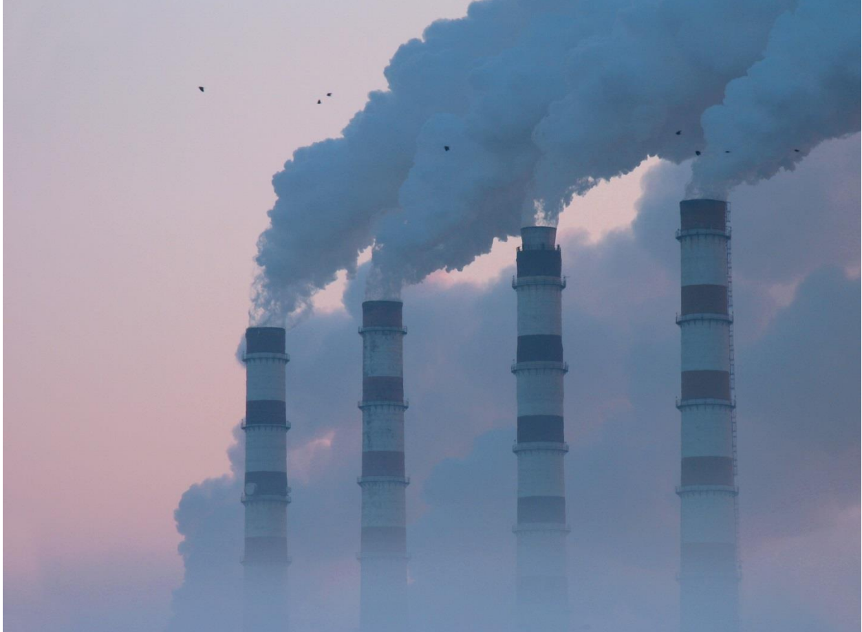
Smoke stacks. Photo by stock.xchng
