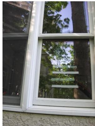
patterns on inside surfaces. Most retrofit solutions are applied to 'side one' but the glass industry has only recently begun marketing 'side one' glass (see database of bird-friendly materials). The photos above show black and white stripes, on the inside and outside of a piece of window glass. It is not surprising that the external white stripes, which reflect the most light, are
