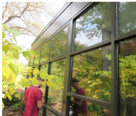
Solyx Bird Safety film covers the entire glass surface of this building at the Bronx Zoo. Photo: Chris Sheppard
