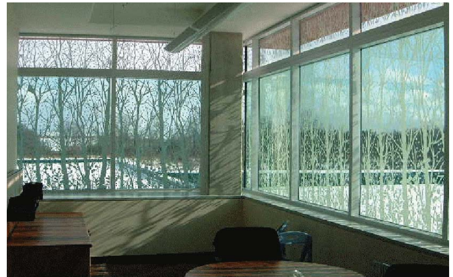
Image 27: The window film is patterned in the shape of trees and attached to the windows of the Earth Rangers Centre in Woodbridge, Ontario. FLAP Toronto collaborated with Earth Rangers to help make their new LEED building safe for birds. The design received an "innovation" LEED credit for addressing bird-building collision issue in the design.
