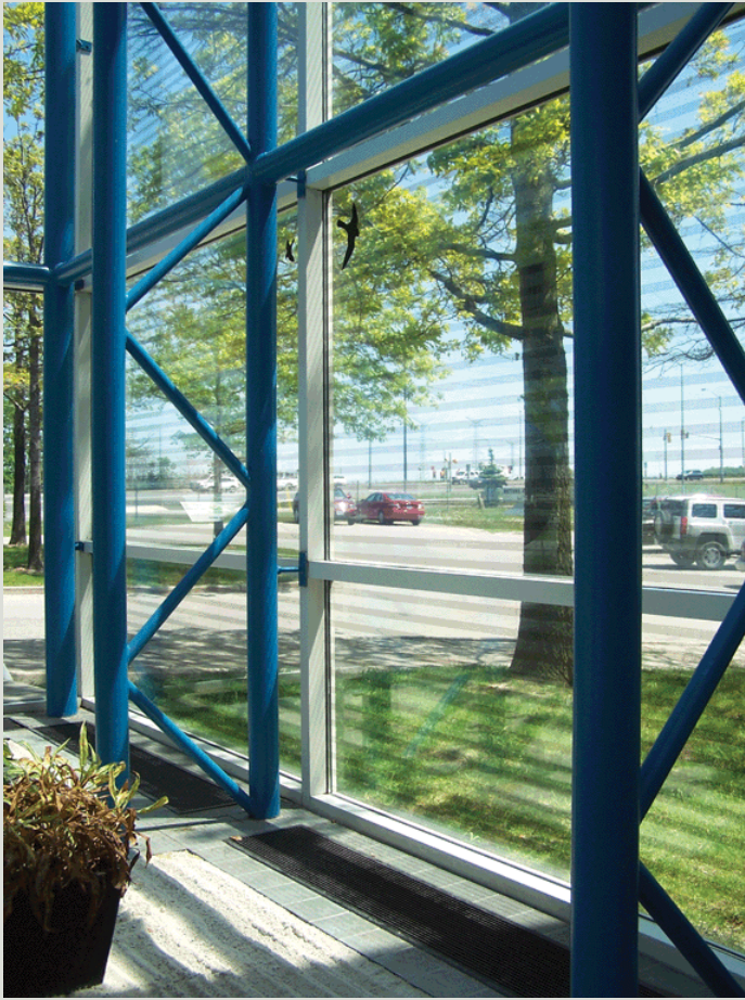
Image 29: A window film applied to the solarium entrance of a town building in Markham, Ontario to prevent bird-window collisions
