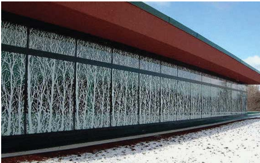
Image 27: The window film is patterned in the shape of trees and attached to the windows of the Earth Rangers Centre in Woodbridge, Ontario. FLAP Toronto collaborated with Earth Rangers to help make their new LEED building safe for birds. The design received an "innovation" LEED credit for addressing bird-building collision issue in the design.
