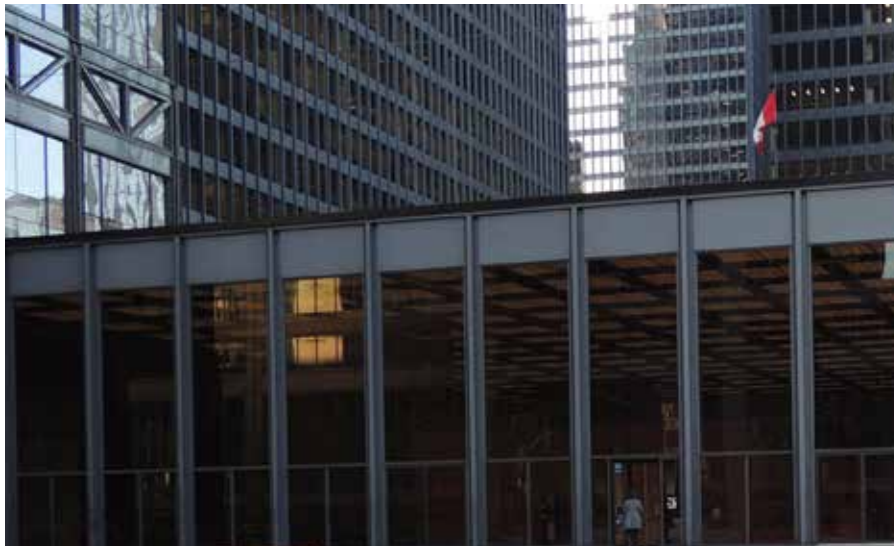
Unacceptable to use Tinted Glass
