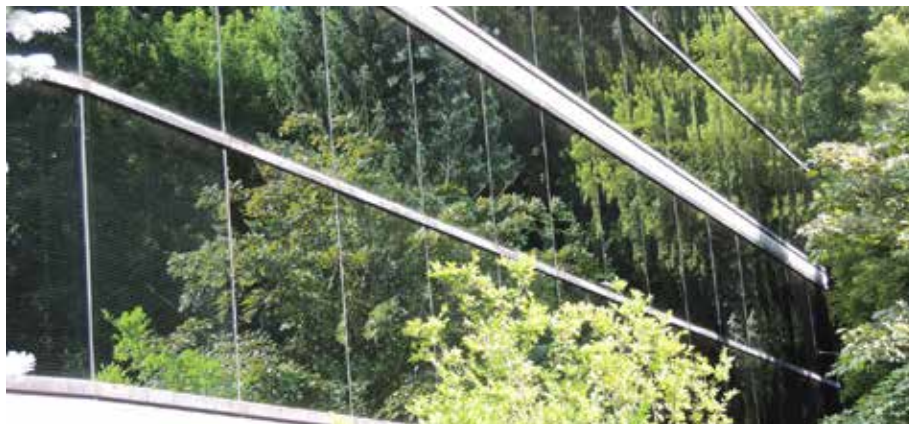
Vegetation and reflective windows create a hazardous environment for birds.
