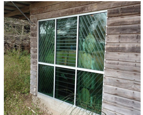
ABC Birdtape, shown here on a window at the Estero Llano Grande State Park, Texas, can be applied in strips or blocks. Photo: Kate Sheppard
