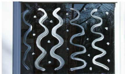
Tempera paint is a washable, long-lasting, and non-toxic solution to preventing bird/window collisions.
