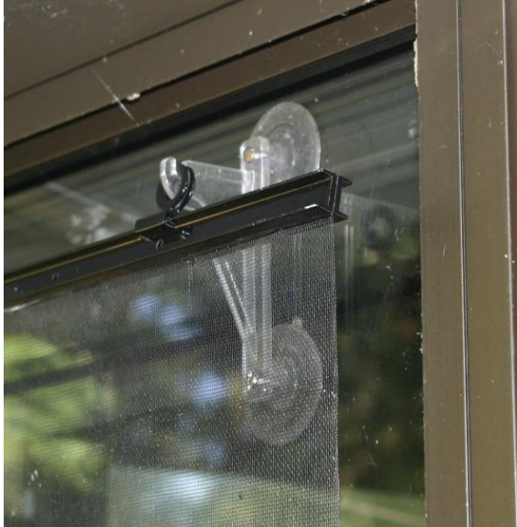
Figure 46. Suction cup mounting for Bird Screens. Photo: BirdScreen.com
