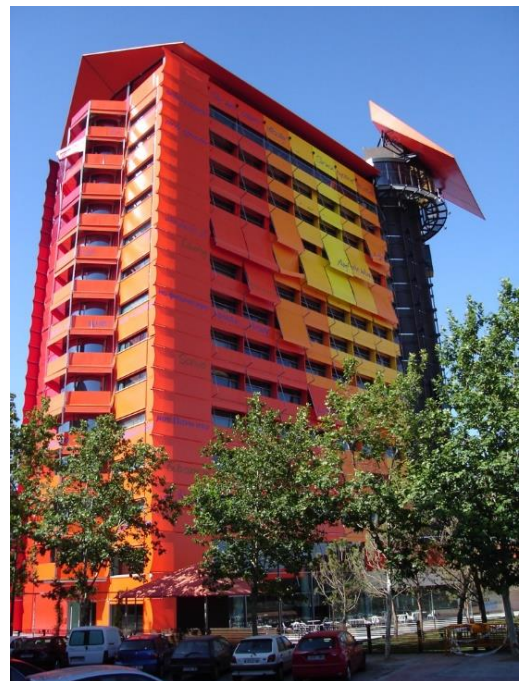
Figure 69. External shades on Hotel Puerta Americas, Madrid, Spain. Photo: Spanaut (Flickr Commons).
