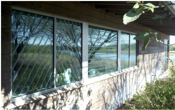
Figure 35. ABC BirdTape at Estero Llano Grande State Park, TX. Photo: Katherine Sheppard
