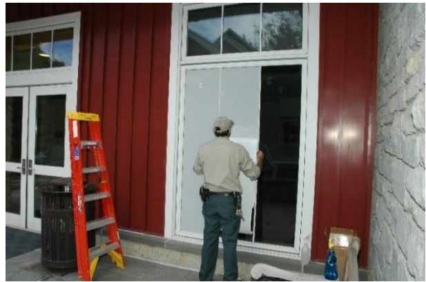
Figure 51. Installing CollidEscape at the National Conservation Training Center. Photo: NCTC
