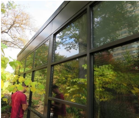
Figure 62. Horizontal Bird Strike film at the Wildlife Conservation Society. Photo: Christine Sheppard
