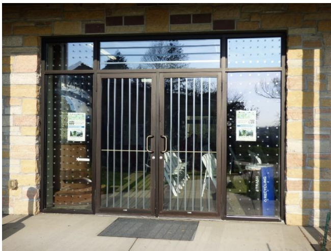
Figure 37. ABC BirdTape at the Carpenter Nature Center, Minnesota. Photo: Joanna Eckles
