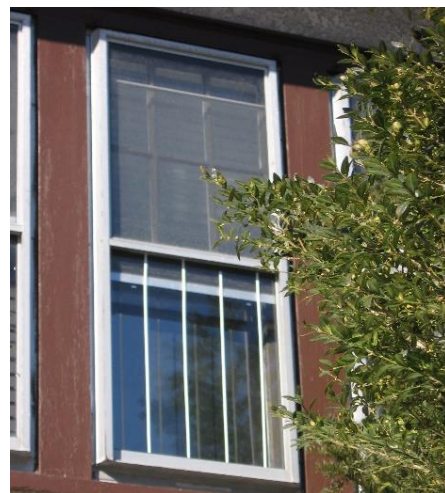
Figure 38. Chart tape stripes on double hung window section without screen. Photo: Christine Sheppard
