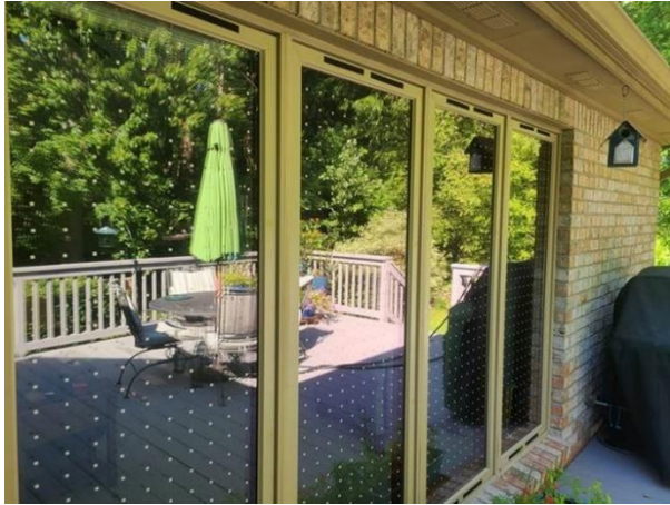
Figure 39. Feather Friendly applied to glass exterior. Photo: Feather Friendly
