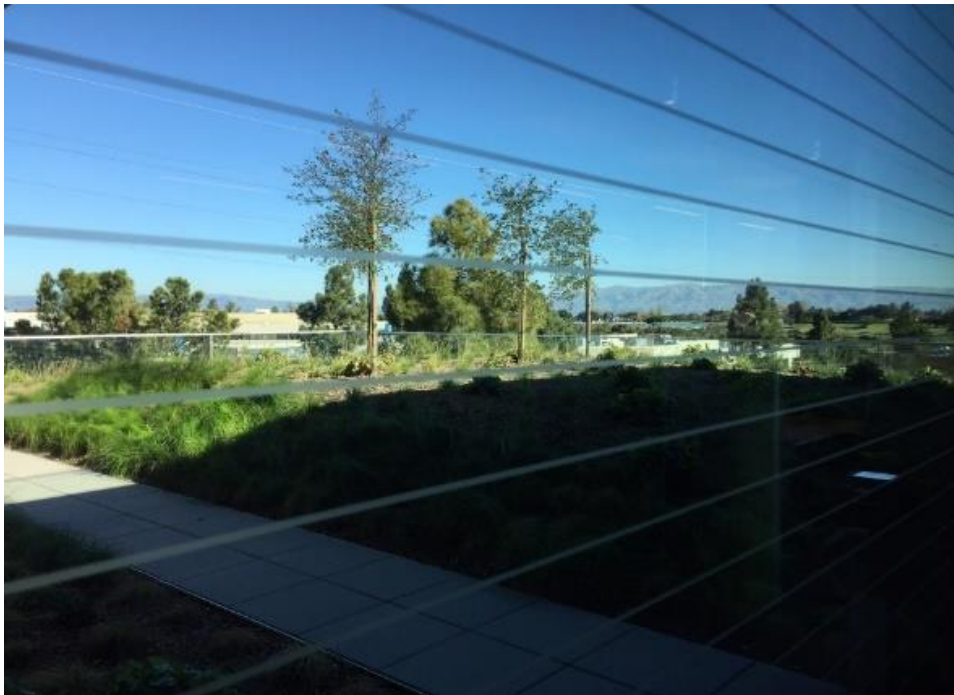
Figure 16. Bird-friendly glass with a frit pattern. Photo: Lila Kakut
