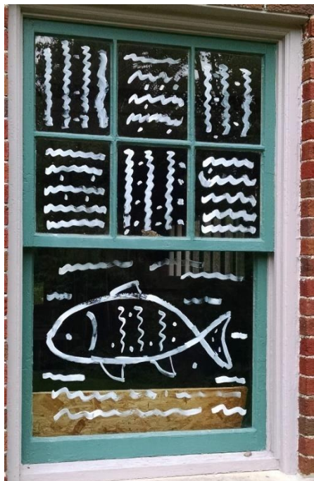
Figure 20. Freehand tempera paint. Photo: Gail Walter
