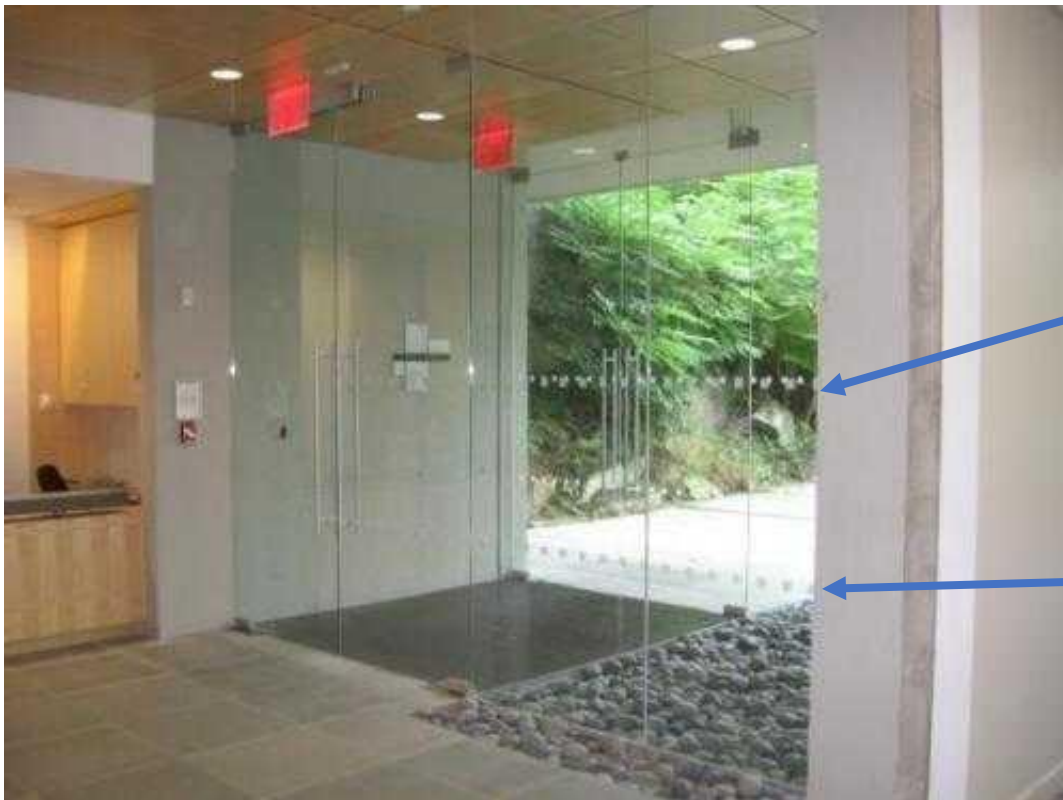
Figure 5. Door with rows of decals required by code. Photo: Christine Sheppard
