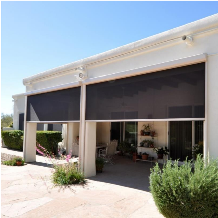
Figure 67. Motorized external solar shades on a private residence. Photo: Donaldson Motorized Shades
