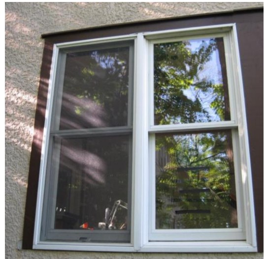
Figure 44. Compare reflection on screened window at left, with unscreened window at right. Photo: Christine Sheppard
